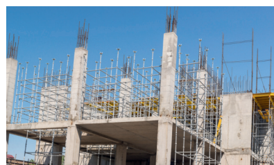
STRUCTURAL AUDIT & HEALTH ASSESSMENT SERVICES
